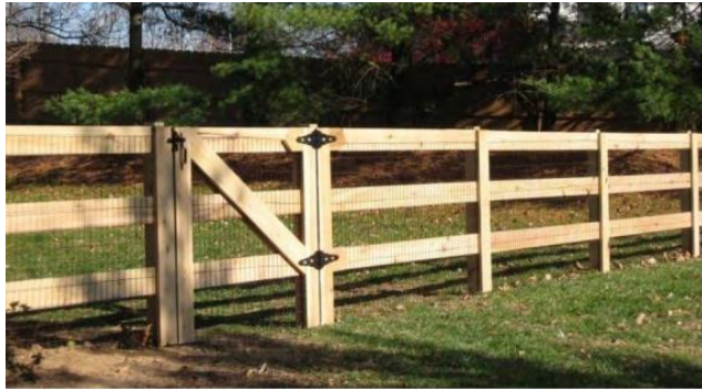
Figure 1109-B: Example of where wire fencing has been mounted on the interior of an approved three-rail fence.
