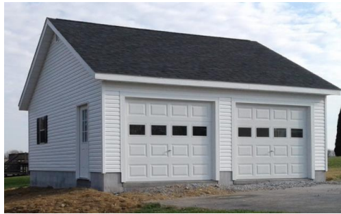
Figure 1117-H: Example image of a detached garage.
