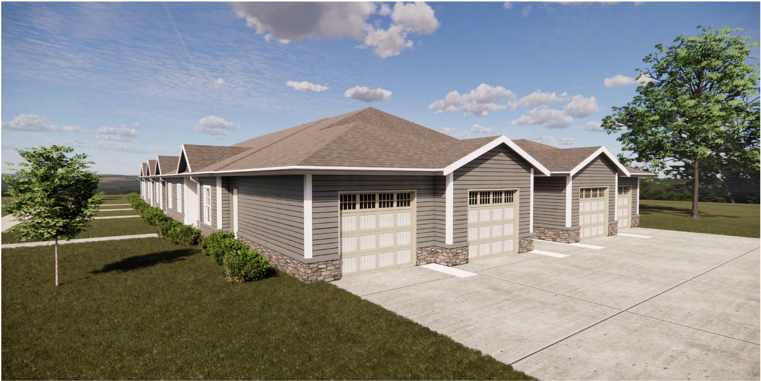
APARTMENTS - (8) UNIT END VIEW
