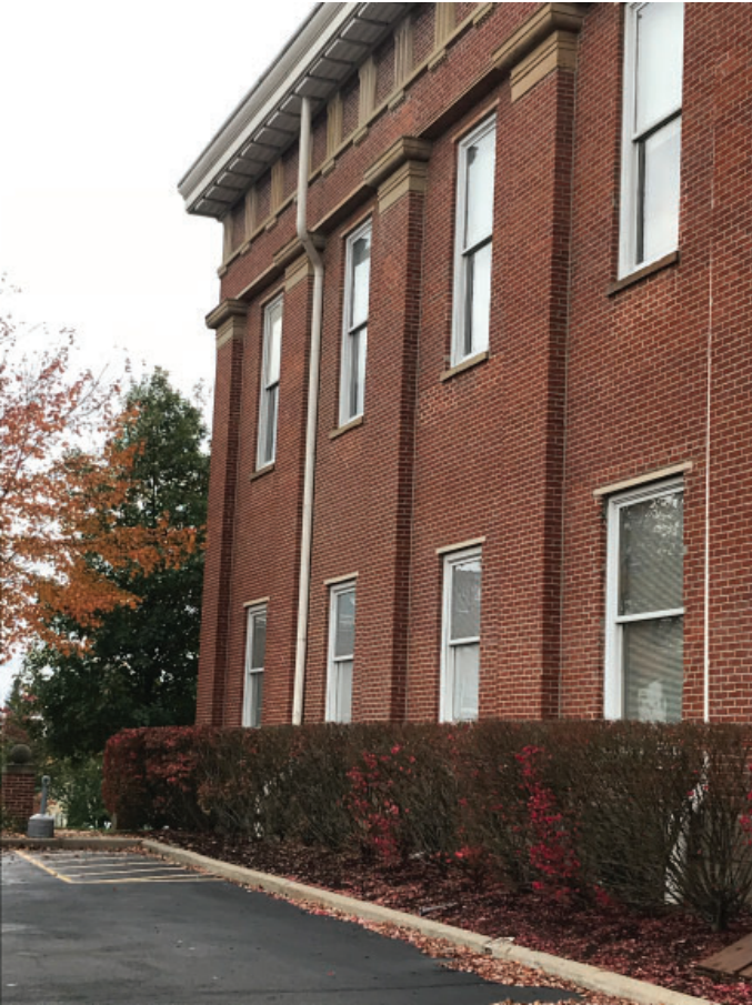
Due to the historic nature of both the front and rear facade, adding a ramp to either would be inauthentic and unwise. A ramp that enters from the side and adjoins the security checkpoint is the best way forward.
