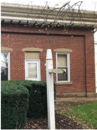
unused sign post
