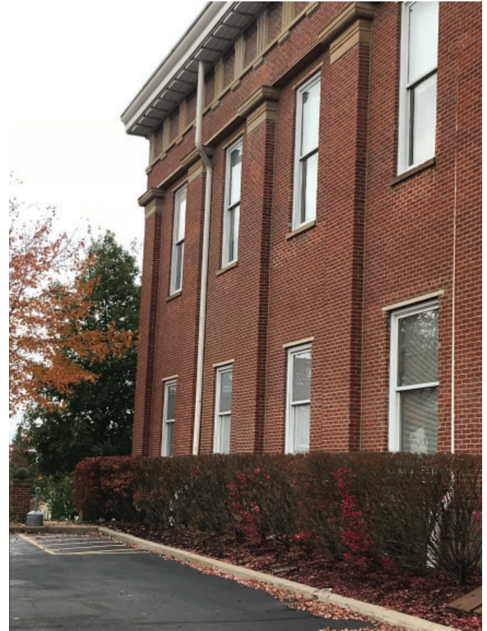
Due to the historic nature of both the front and rear facade, adding a ramp to either would be inauthentic and unwise. A ramp that enters from the side and adjoins the security checkpoint is the best way forward.
