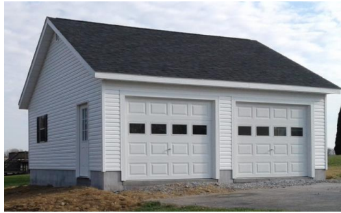
Figure 1117-G: Example image of a detached garage.
