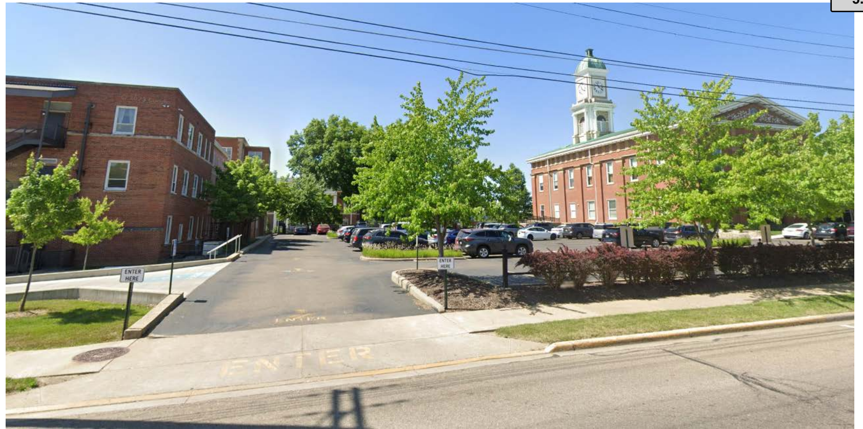
WEST - FACING SOUTH; WEST PARKING LOT
