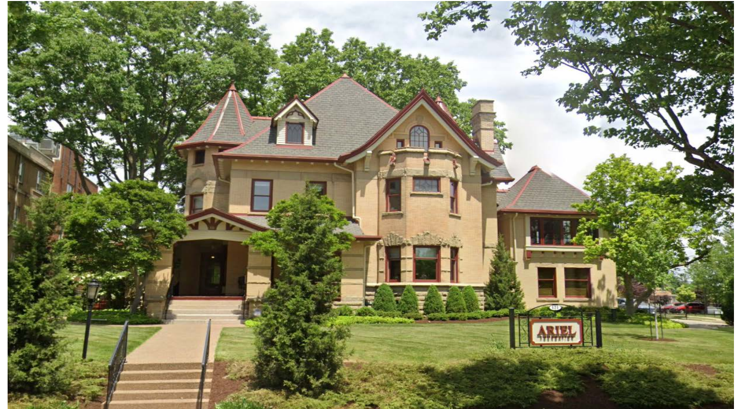
EAST - FACING NORTH FROM HIGH ST.
