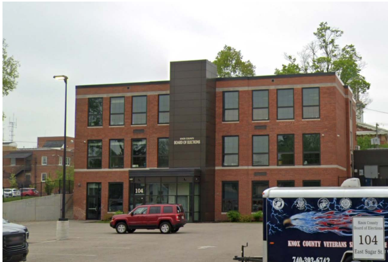
WEST, FACING SOUTH FROM E. SUGAR ST. RENOVATED 2019, METAL PANEL REFERENCE.
