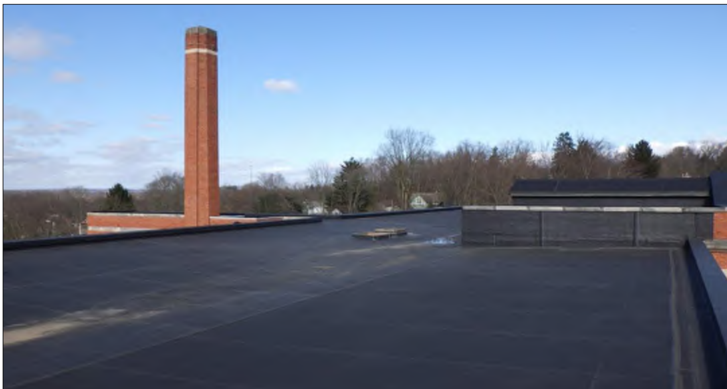
Photo 8: Overall view of roof, looking northwest.
