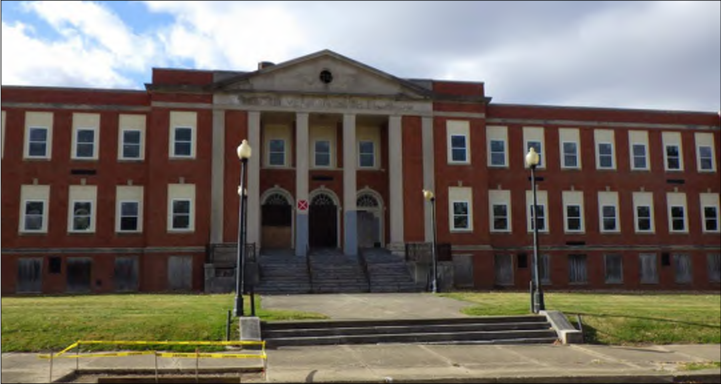
Photo 1: East (front) elevation of the building.
