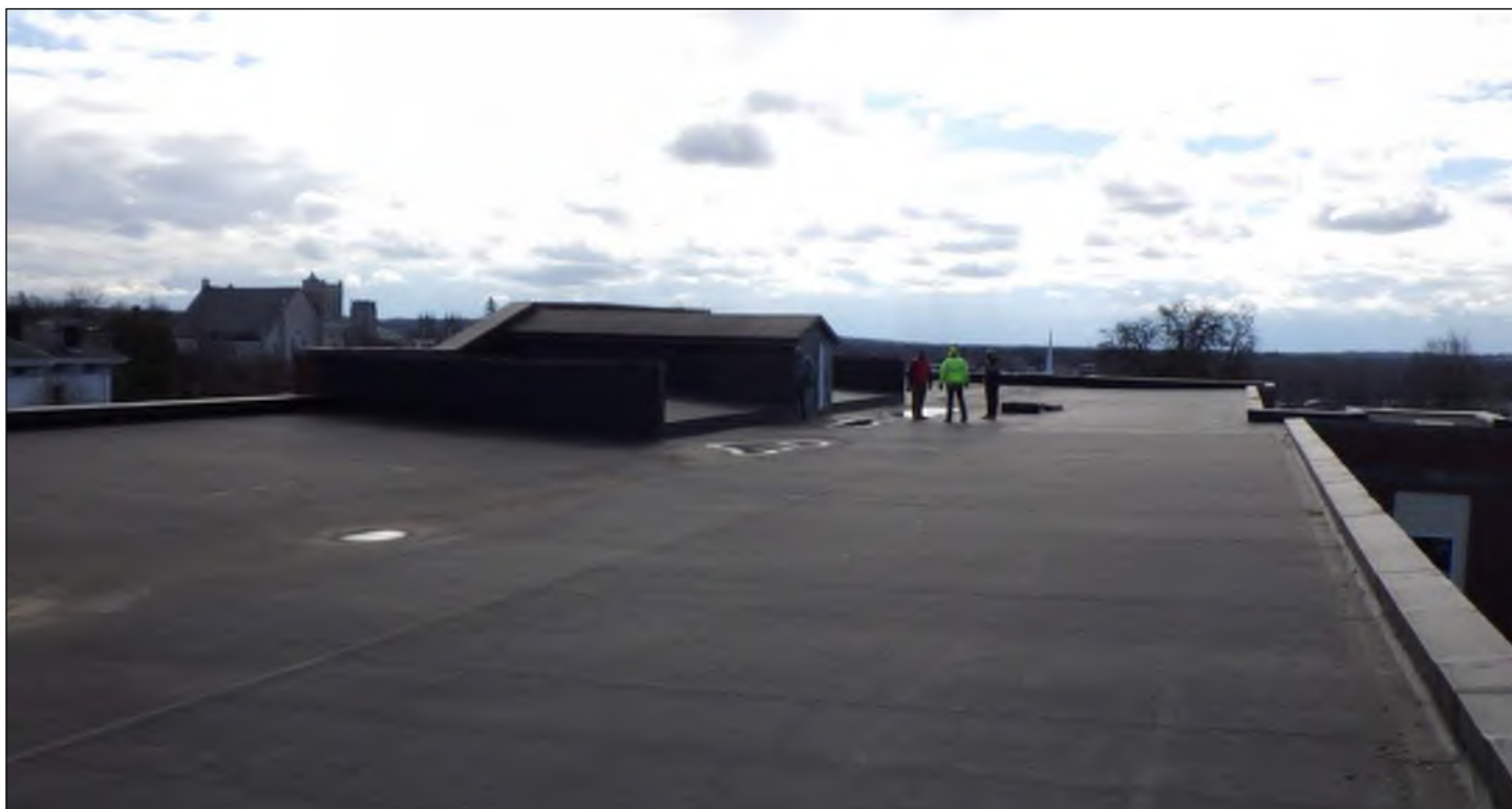
Photo 10: Overall view of roof, looking southeast.
