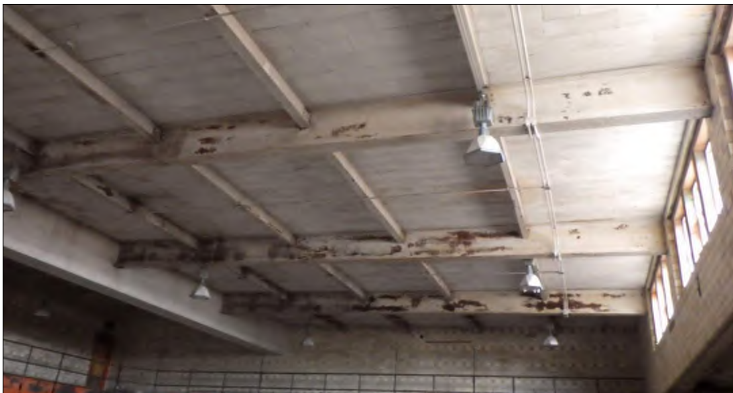
Photo 58: Overall view of steel beams supporting the gymnasium roof, looking south.
