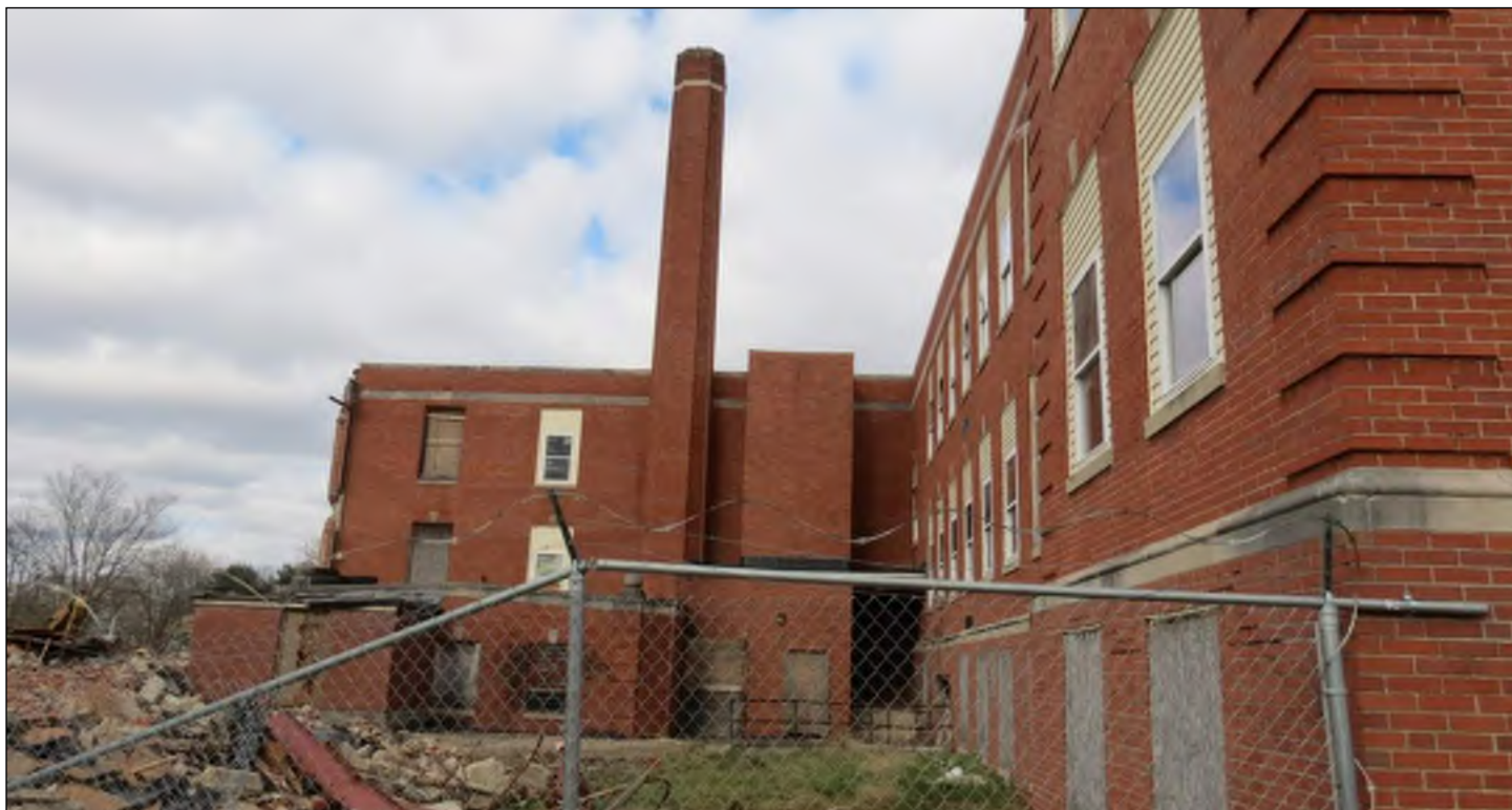
Photo 5: West (rear) elevation of the building.
