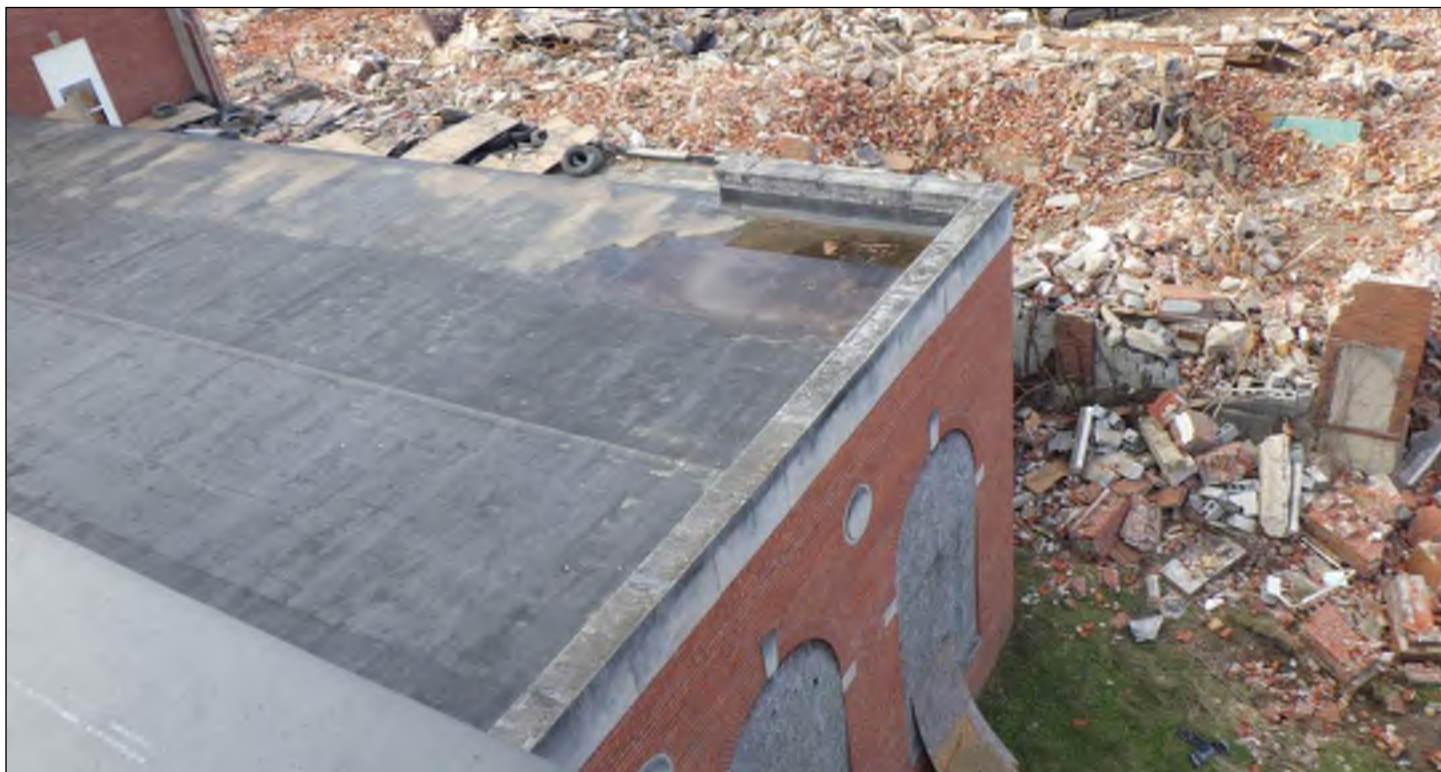
Photo 13: Overall view of high gymnasium roof, looking southwest.
