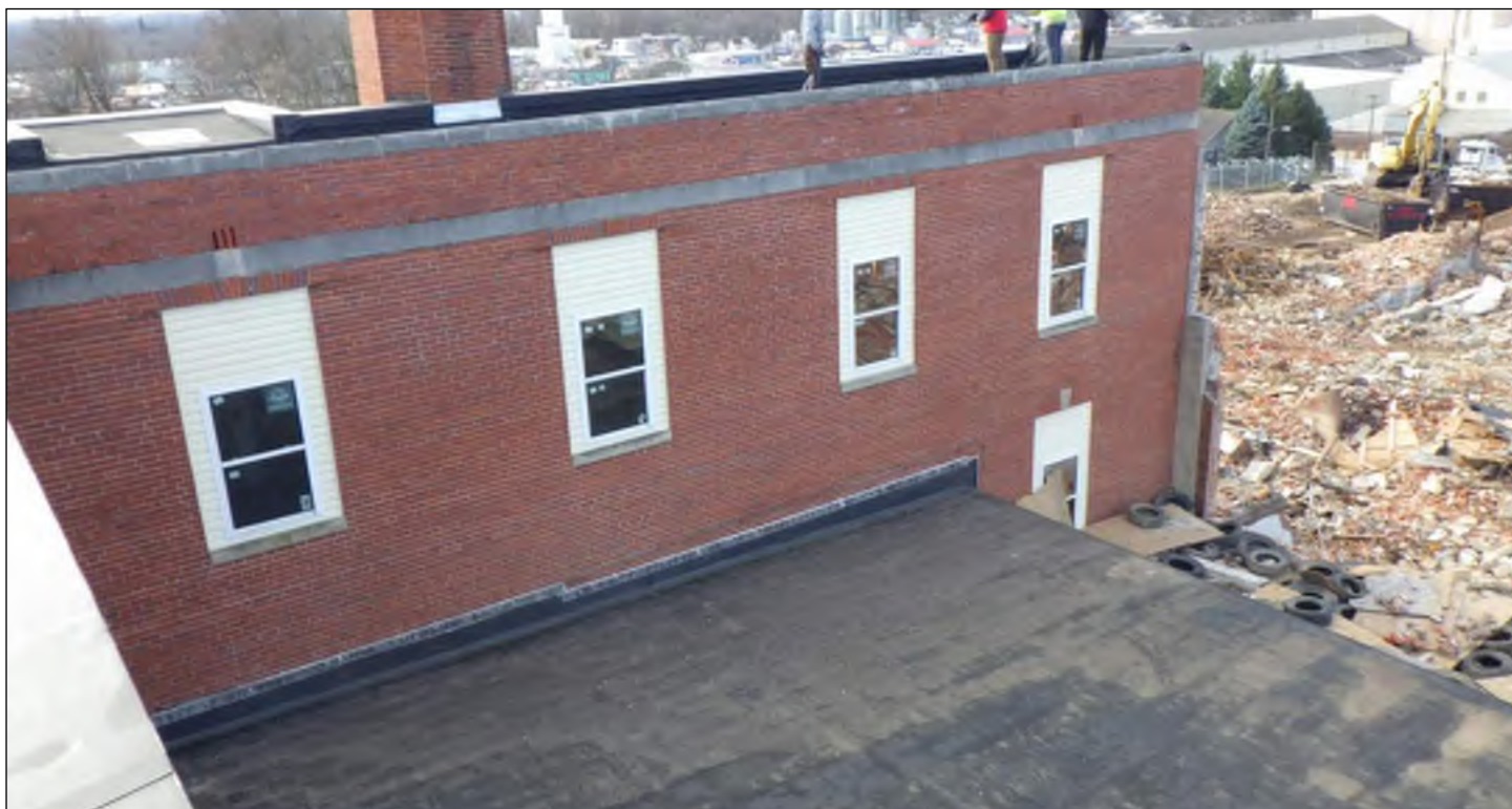
Photo 14: Overall view of high gymnasium roof, looking southwest.
