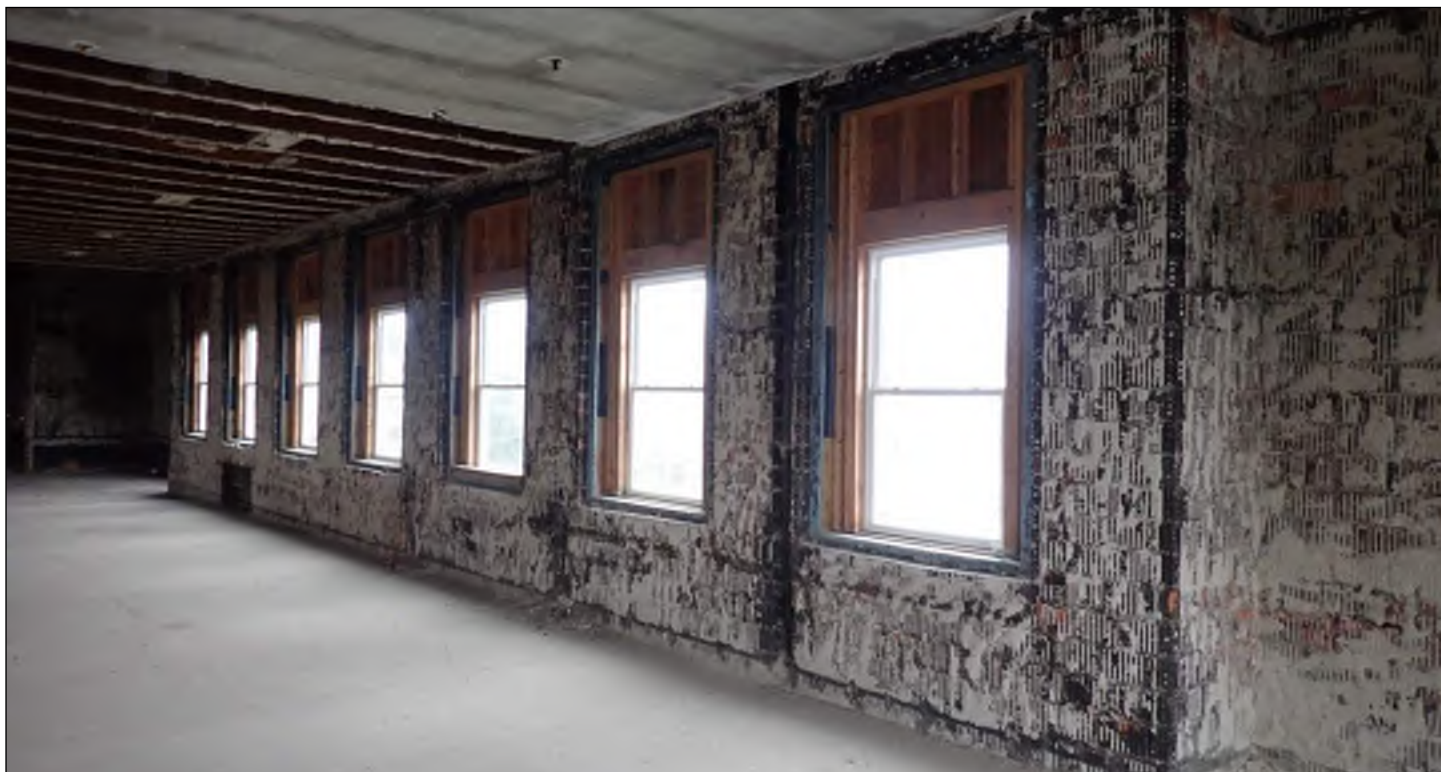
Photo 53: Brick masonry bearing wall interior .
