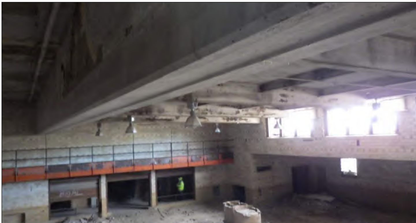
Photo 61: Close-up view of concrete-encased bottom flange of built-up steel plate girder.
