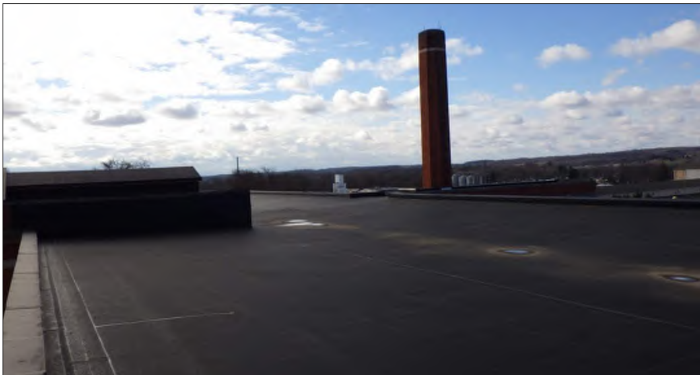
Photo 9: Overall view of roof, looking southwest.
