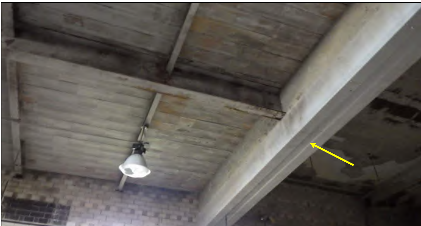
Photo 60: Steel plate girder (obscured from view by finishes) (arrow).
