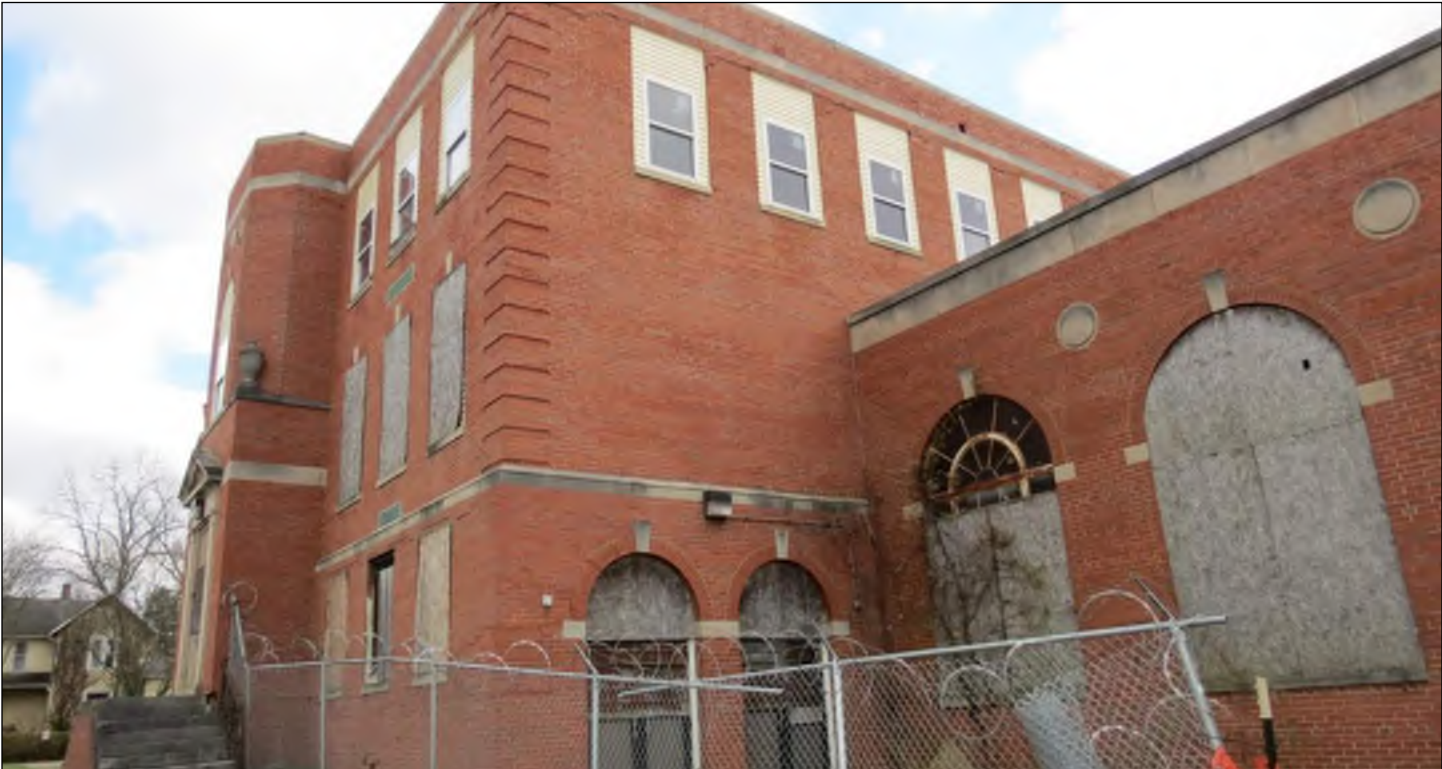
Photo 4: West (rear) elevation of the building.
