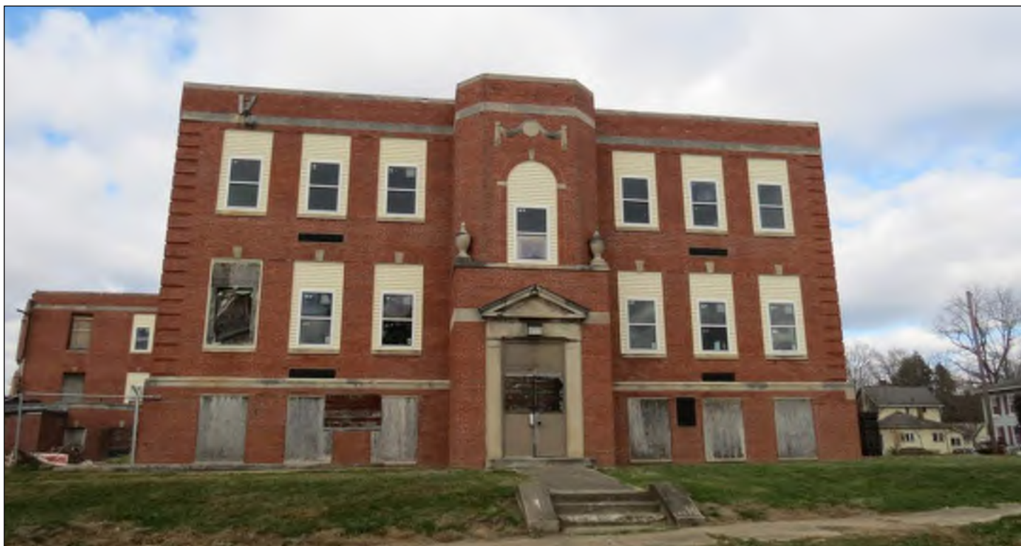
Photo 6: South (side) elevation of the building.
