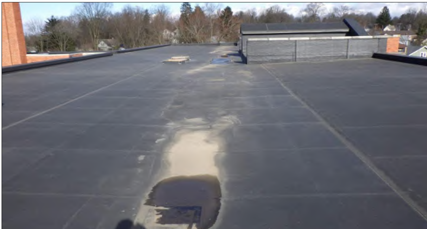
Photo 7: Overall view of roof, looking north.
