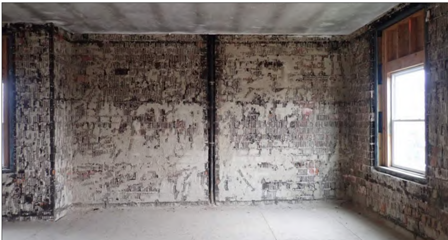
Photo 54: Brick masonry bearing wall interior.
