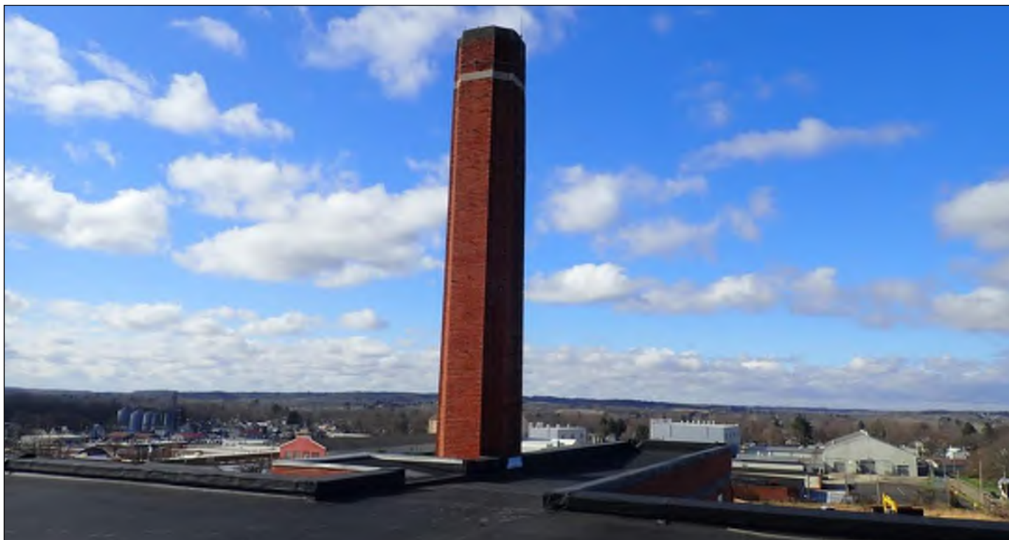
Photo 17: Overall view of smokestack, looking southwest.
