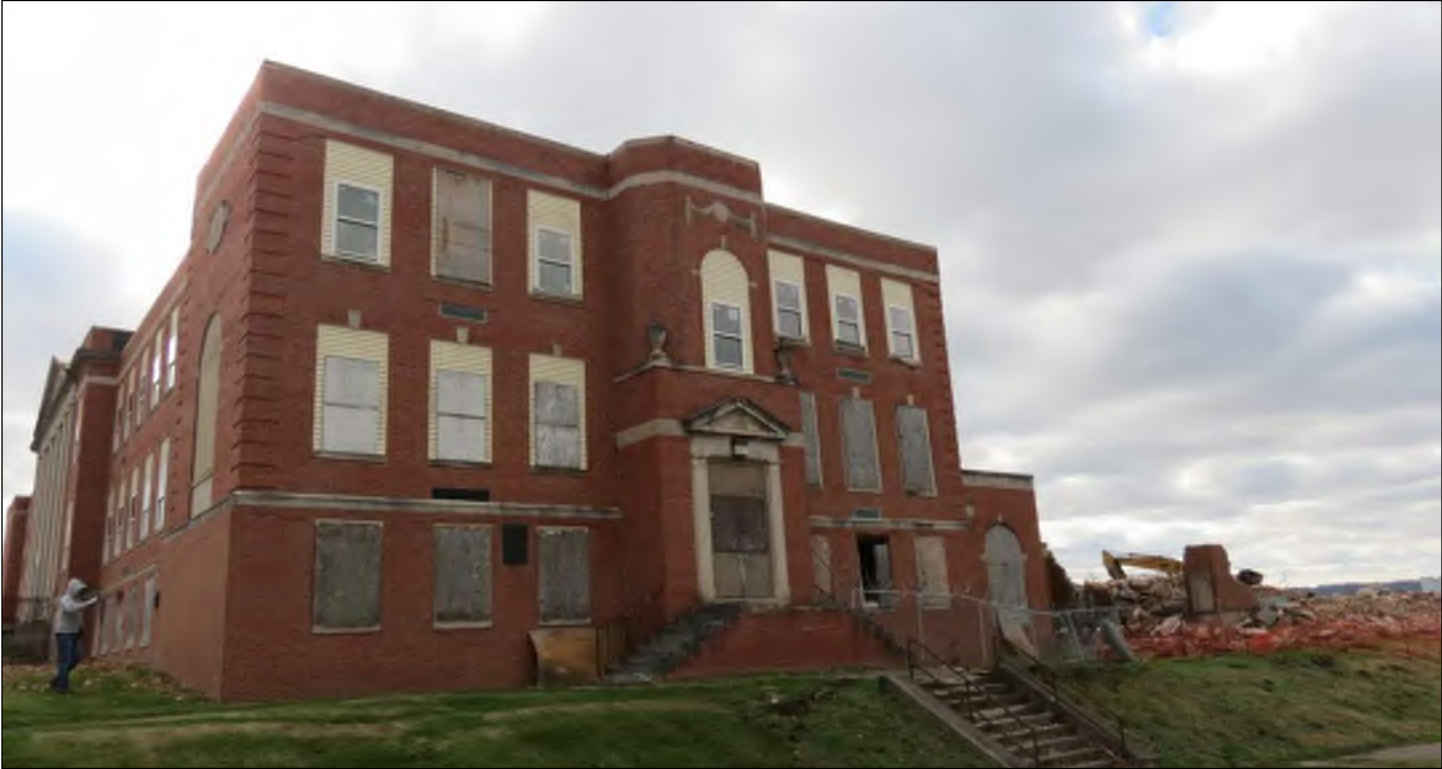
Photo 3: North (side) elevation of the building.
